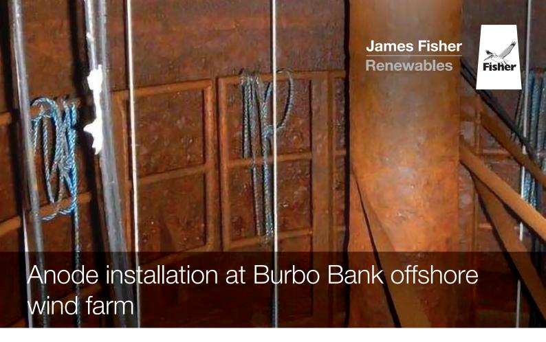
James Fisher Marine Services\* installed Cathodic Protection across 25 individual assets located at Burbo Bank, an offshore wind farm operated by Dong Energy – now Ørsted.
